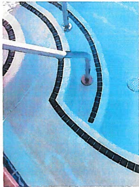
Staining & pitting of Plaster
