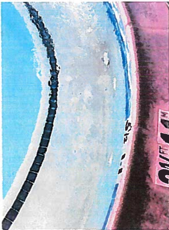
Staining & pitting of Plaster
