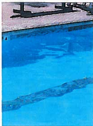
Blue Tiles that have been replaced due to the old tiles failing and falling out
