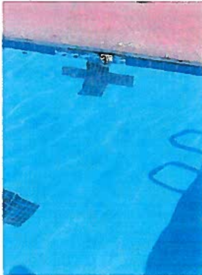
Blue Tiles that have been replaced due to the old tiles failing and falling out
