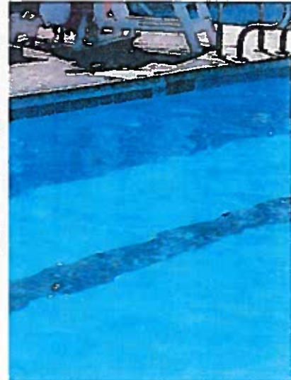
Blue Tiles that have been replaced due to the old tiles failing and falling out
