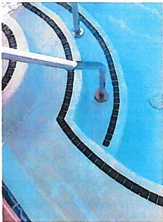
Staining & pitting of Plaster
