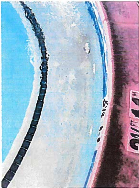
Staining & pitting of Plaster
