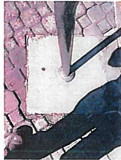
Blue Tiles that have been replaced due to the old tiles failing and falling out
