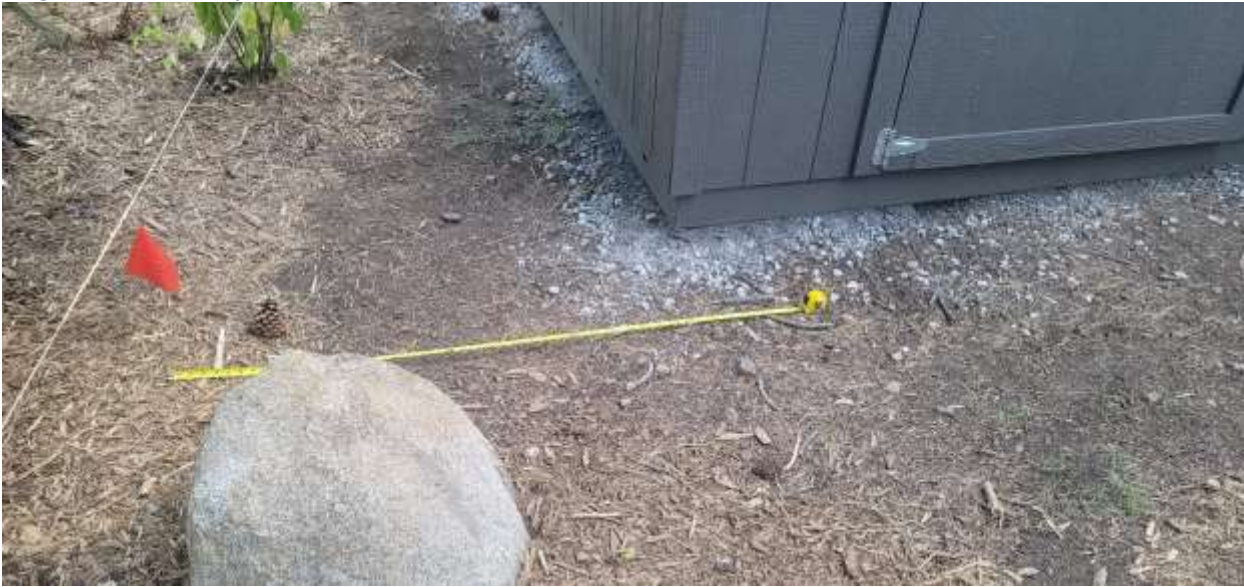
Image 2: Front corner of shed approximately 8 inches into 5' setback
