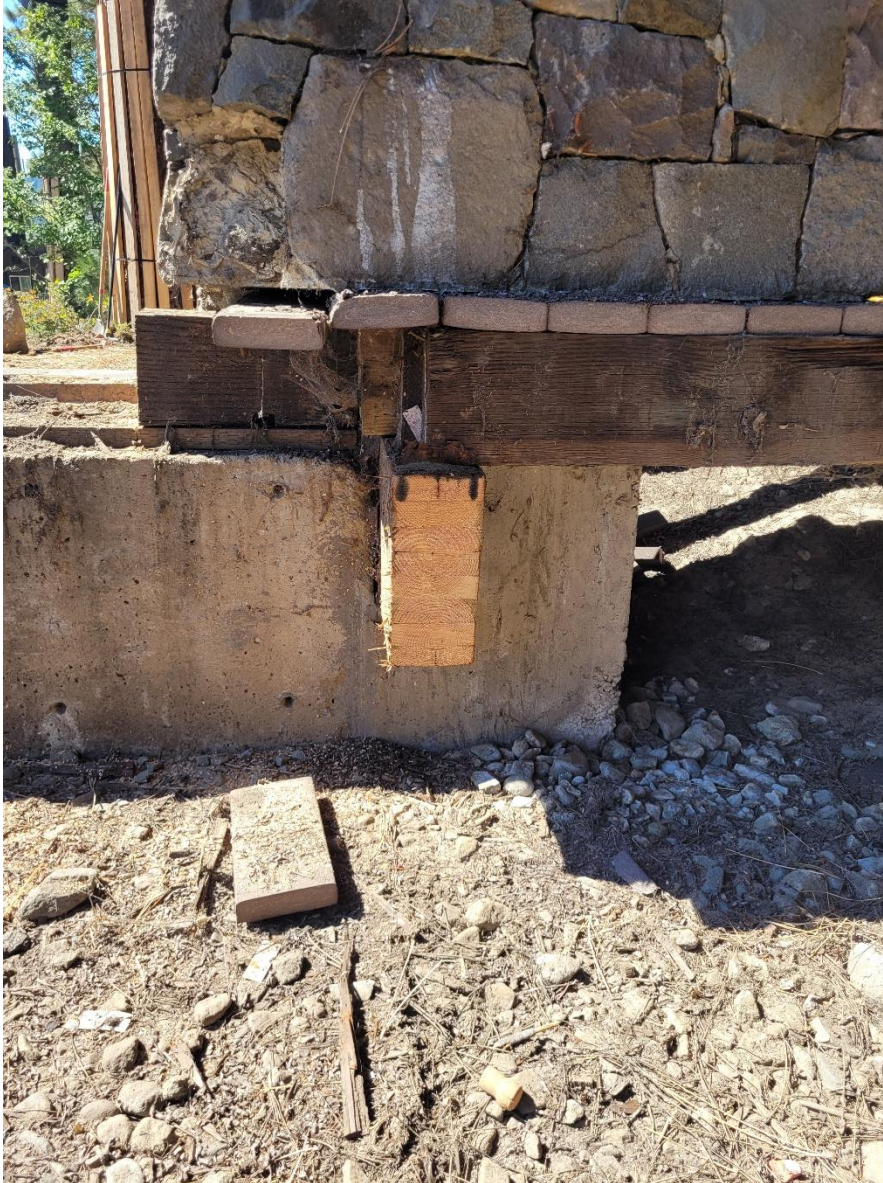
Stone veneer resting on Trex decking
